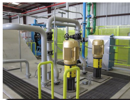
240 GPM (912 LPM) Filter System for 2-Wire Rod Breakdown Machine
